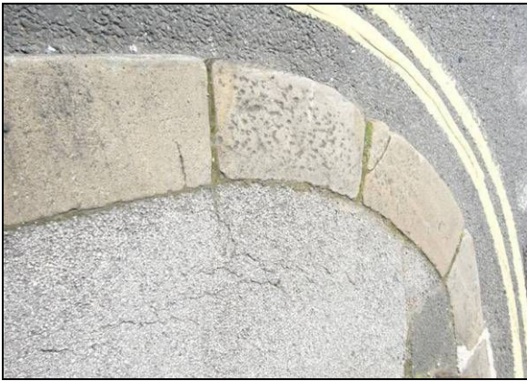
Historic stone kerb
