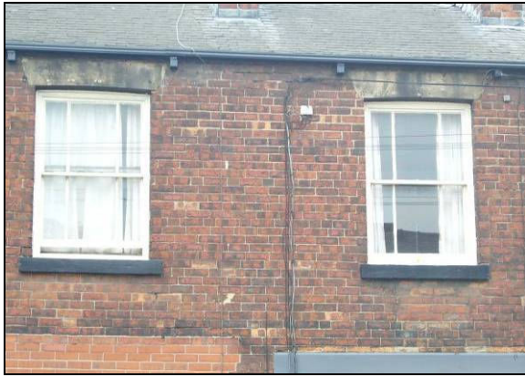
Sash-windows with margin lights
