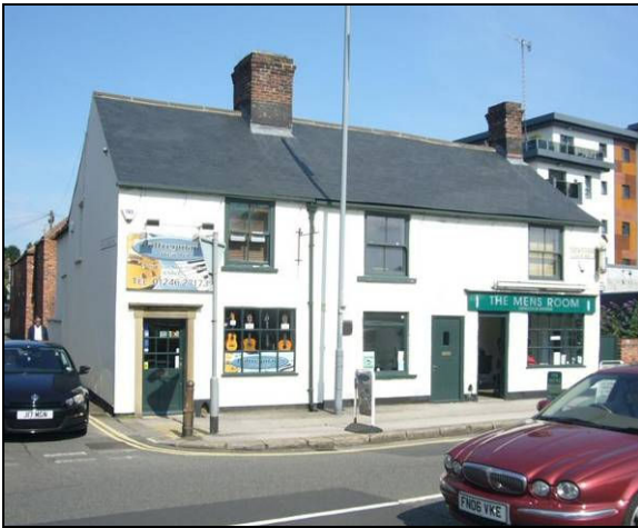
Nos. 169 & 171 Chatsworth Road
