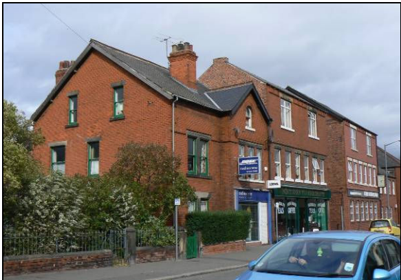
Red brick buildings
