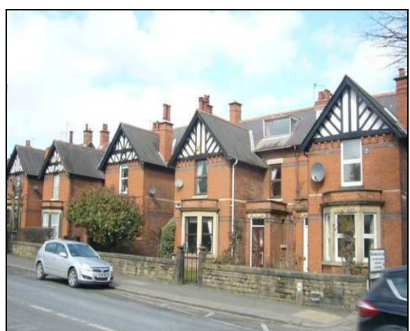
Nos. 485-497 Chatsworth Road
