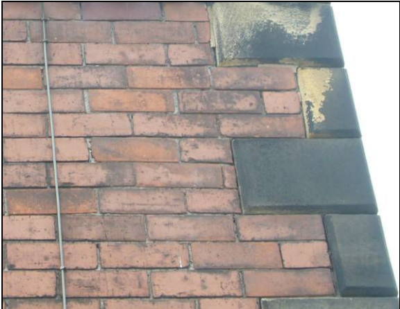
Stone quoins on brick wall
